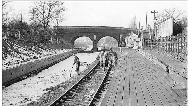
Above: Contrasts at Mill Hill The Hale, before work had started (Left) on electrification and track doubling with N2 4738 with articulated coaches working from Edgware to Finchley. After the service had been suspended (Right), the second platform is under construction and the alignment made for the future northbound track. The wooden platform on the right appears to be unaltered at this stage.
