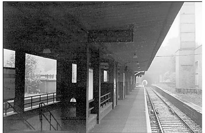
A view on a murky day of Highgate High Level station, north end looking south, after reconstruction by London Transport for the Northern Line from Moorgate (which never came). On the left can be seen the stairs to the deep-level station. Note on the track at bottom right the tripcock testing apparatus for locomotive-hauled trains.
